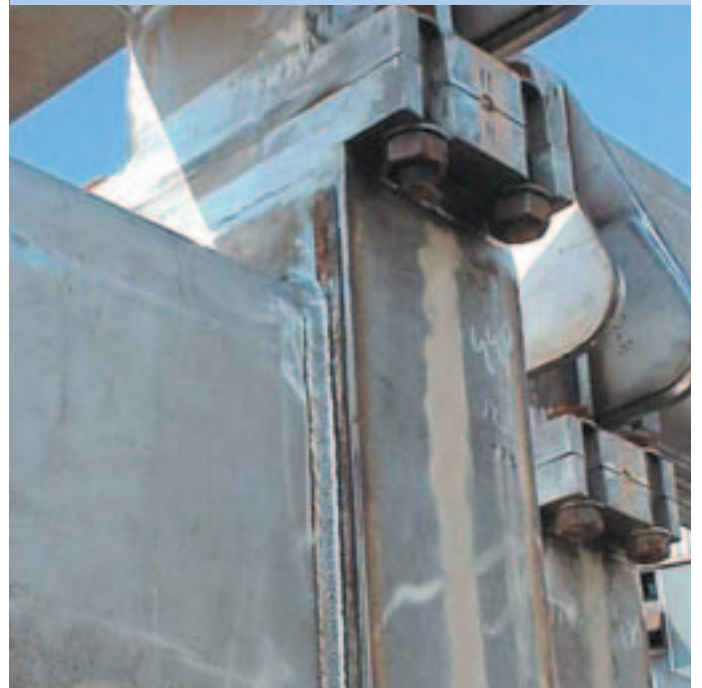
异种钢焊缝， 采用伯乐CN 23/12 Mo PW-FD焊接
